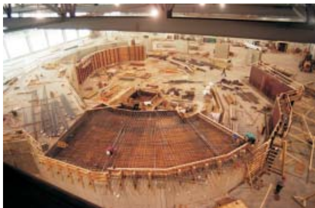
CLS shielding tunnel during fabrication.
