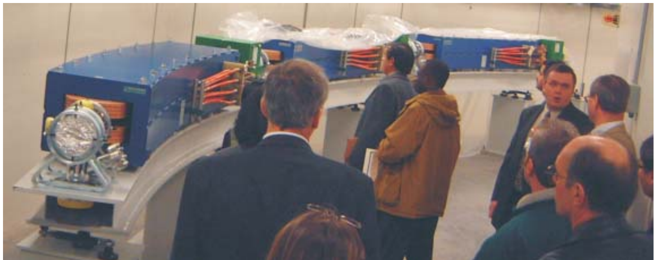
A partially installed section of the CLS booster ring is viewed by a group from the CLS Users' Meeting (Nov. 17, 2001).
