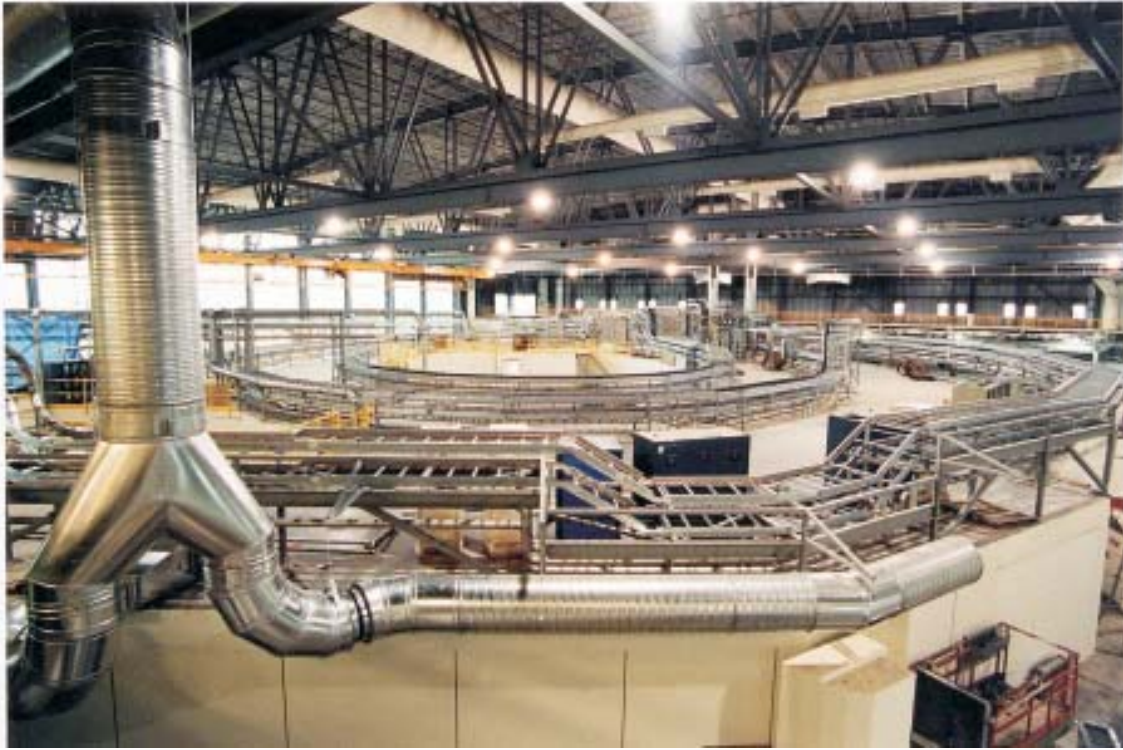
Canadian Light Source under construction (November 2001).
